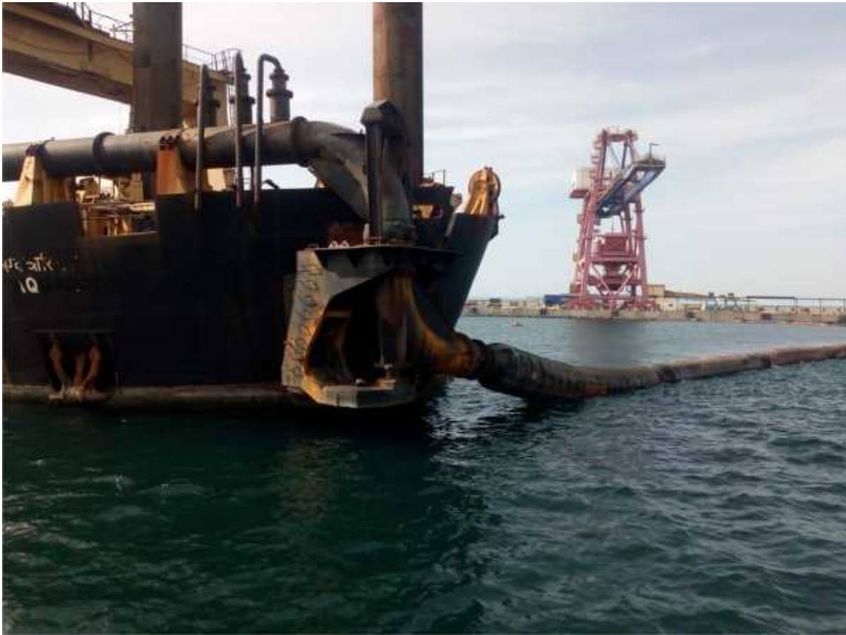
Connection of self floating pipeline with CSD DR-Aquarius
