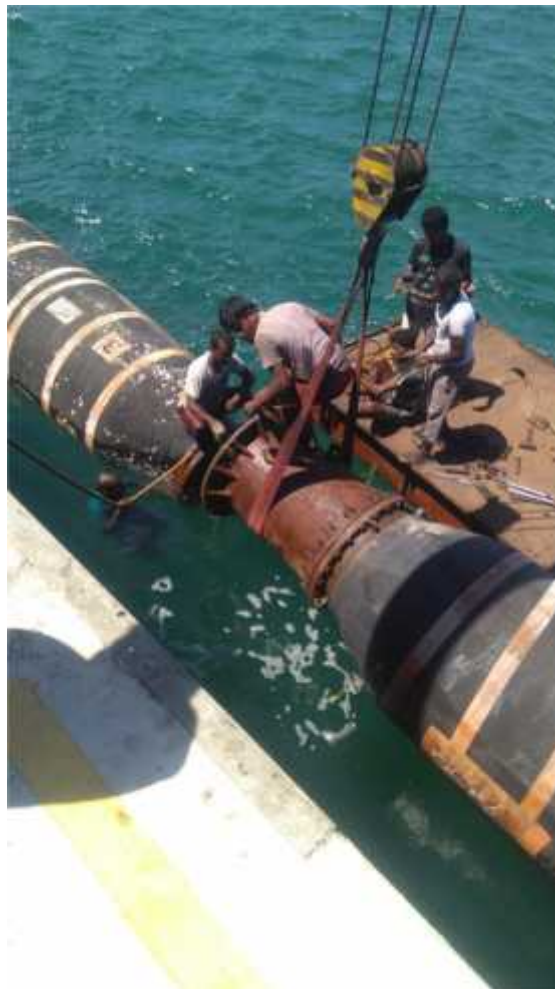
Connecting self floating pipeline
