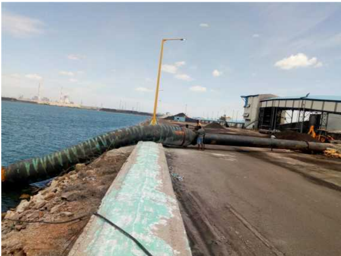
Self floating connected to Shore Pipeline to discharge dredged material
