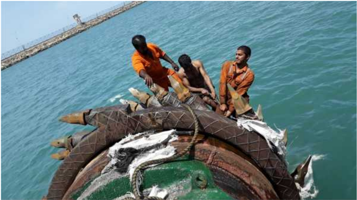
Clearing of underwater obstructions from Cutter teeth
